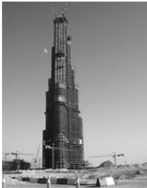
Under construction: the Burj Dubai, the world's tallest building. The actual height is a closely guarded secret and won't be revealed until construction is completed.
